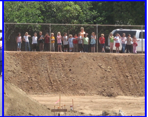
On-lookers at Cajon Park Construction Site
